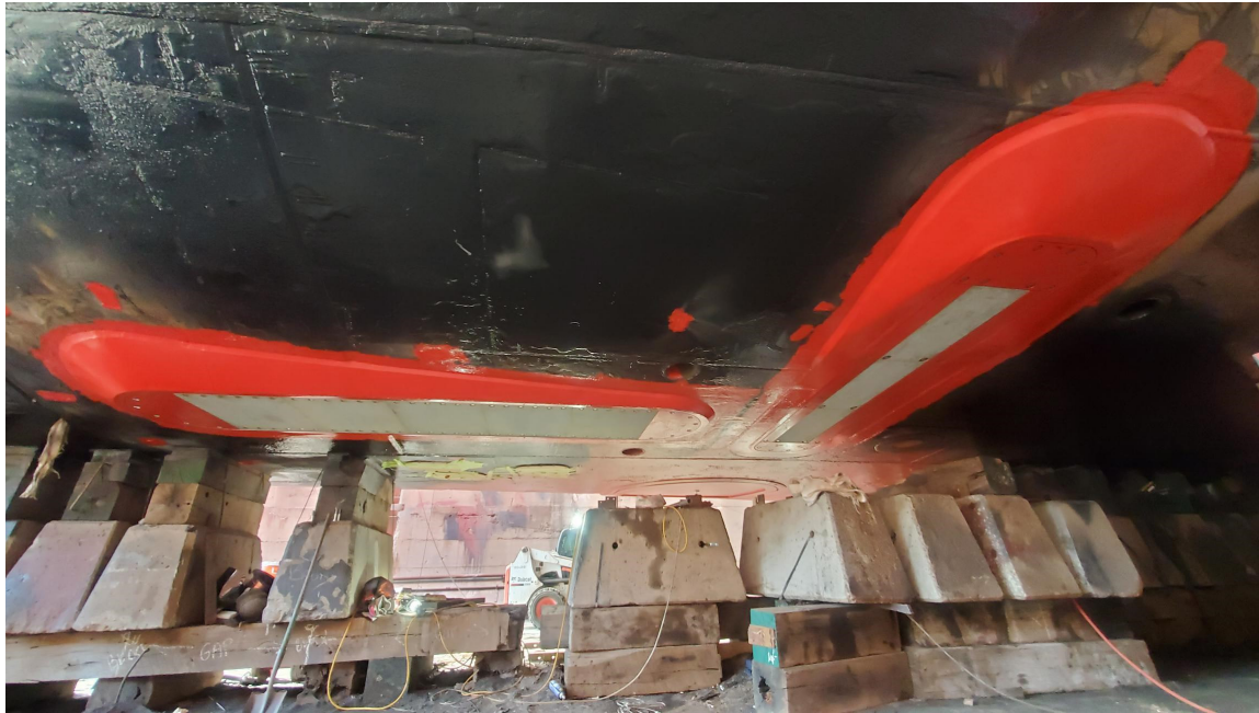
Figure 5-1: EM304 installed on the hull of the CCGS Amundsen
