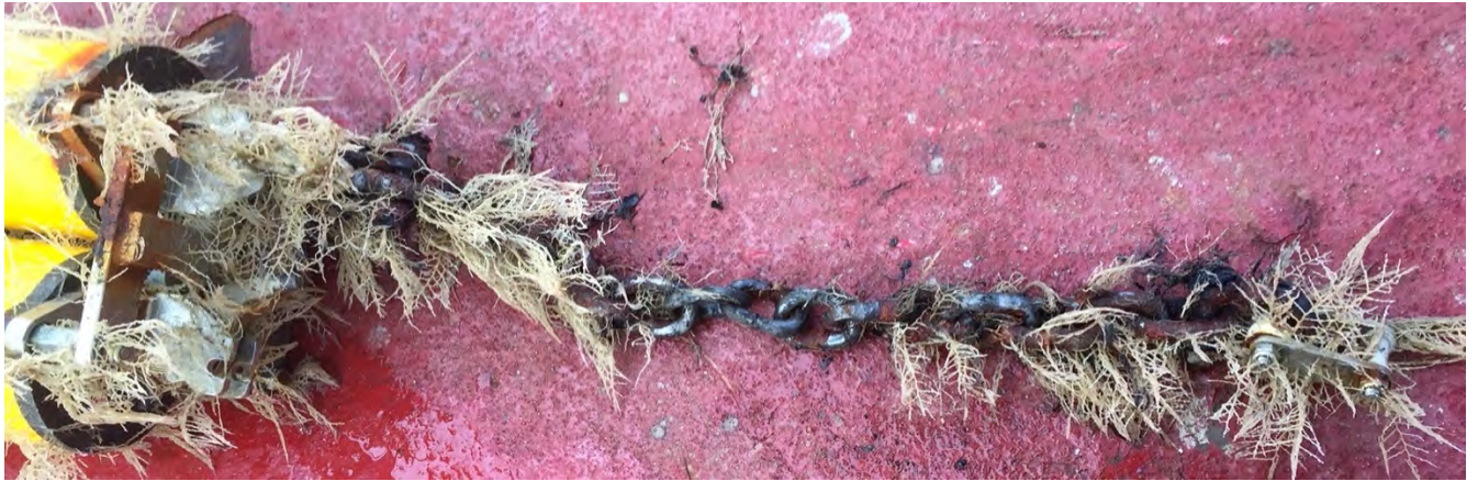
Figure 8-7. Drop ring corrosion from MkB1-20
